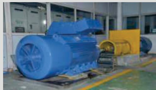
Large Motor Test Facility
