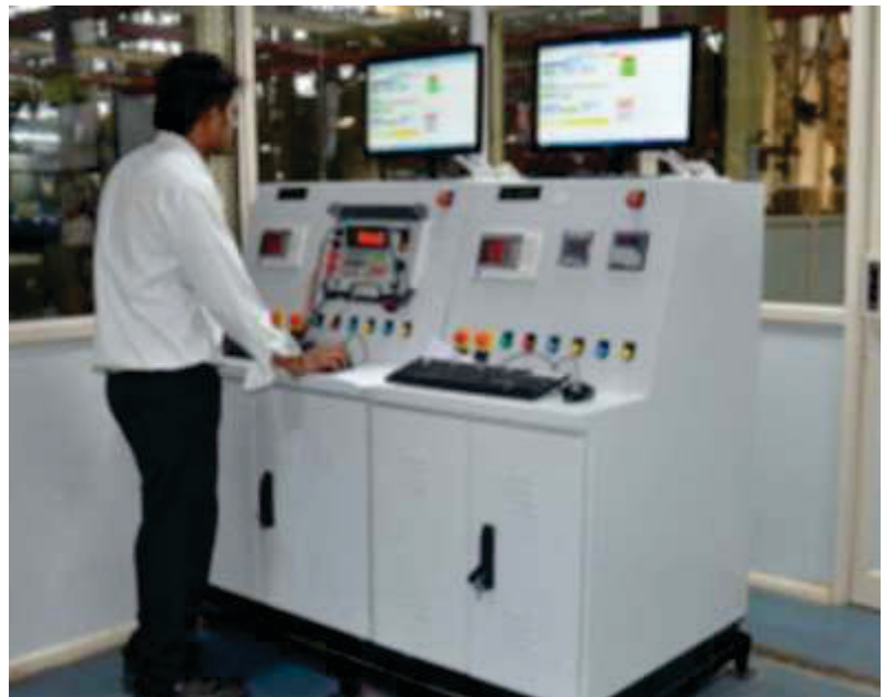
SCADA Test Facility
